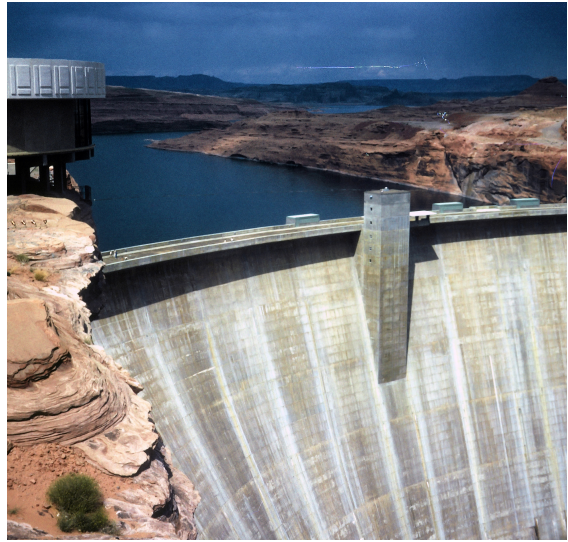
Glen Canyon Dam
