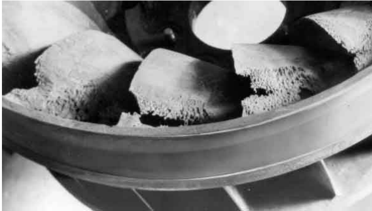
Figure 6.4. Cavitation damage on the blades at the discharge from a Francis turbine.
