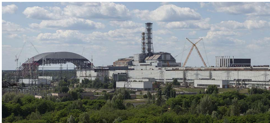
Figure 7.11: Cylindrical entombment structure (left) being prepared for installation over the damaged Chernobyl reactor (center). Photograph reproduced with the permission of the owner, Ingmar Runge.
