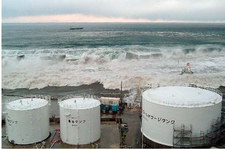
Figure 7.12: Tsunami striking the Fukushima Daiichi nuclear power plant on March 11, 2011. Reproduced with permission of Tokyo Electric Power Company (TEPCO 2011).
