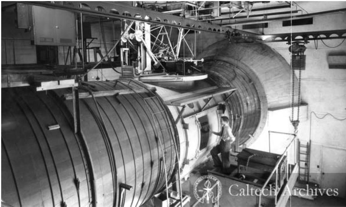
Figure 2: Ten Foot Wind Tunnel at the California Institute of Technology.
