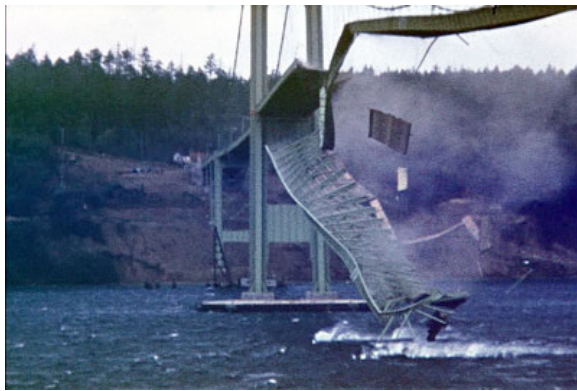
Figure 7: Failure of the Tacoma Narrows suspension bridge as a result of vortex shedding.
