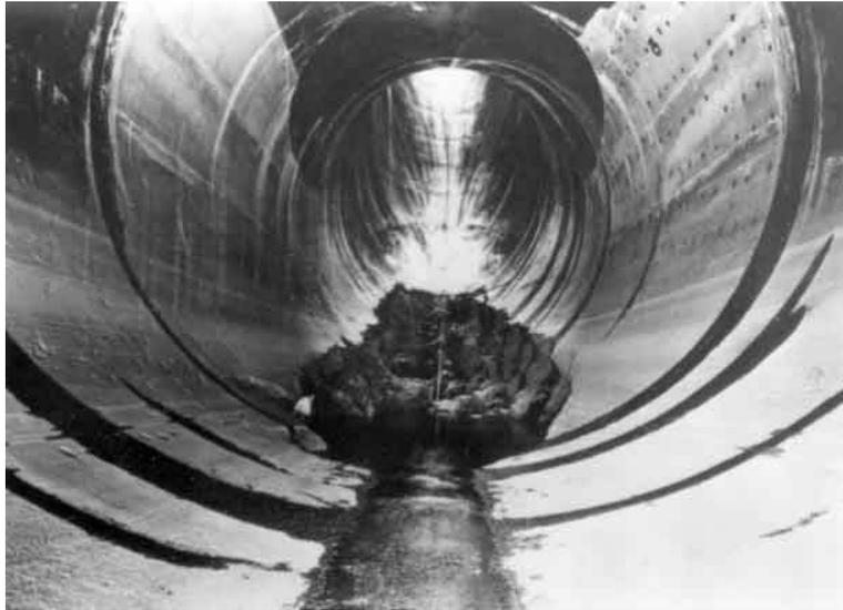
Figure 3: Cavitation damage to the concrete wall of the 15.2 m diameter Arizona spillway at the Hoover Dam. The hole is 35 m long, 9 m wide and 13.7 m deep. Reproduced from Warnock (1945).
