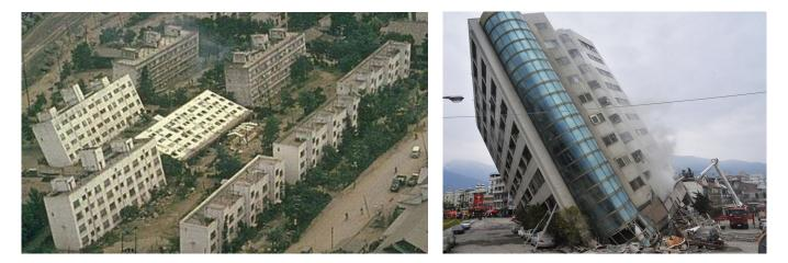
Figure 1: Soil liquefaction: Left: Magnitude 7.5 earthquake, June 1964, Niigata, Japan (Photo: Joseph Penzien.) Right: Magnitude 6.0 earthquake, February 2018, Hualien, Taiwan (Photo: CNA).
