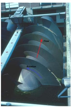
Figure 1: Left: Ancient Persian water wheel. Right: An Archimedes screw used to lift water in Netherlands from one canal to another.
