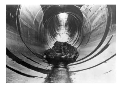
Figure 3: Cavitation damage to the concrete wall of the 15.2 m diameter Arizona spillway at the Hoover Dam. The hole is 35 m long, 9 m wide and 13.7 m deep. Reproduced from Warnock (1945).
